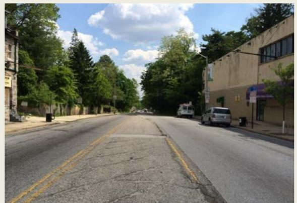
Photo 19: Cracked pavement and faded pavement markings
