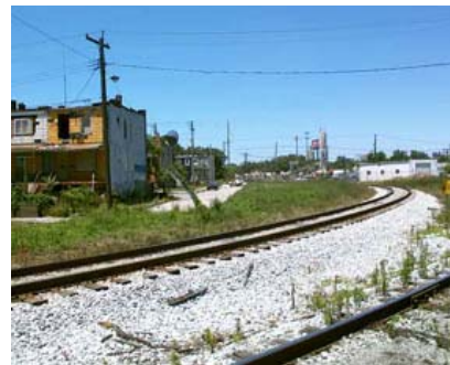
b CSX tracks and buffer parcels
