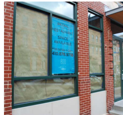
Figure 17. Renovated Space for Lease on Charles Street
