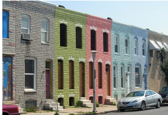
Renovation of row-houses is already underway in the MMF area.
