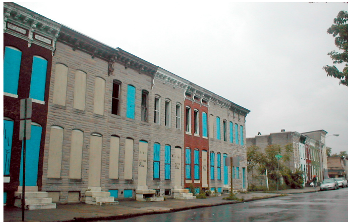
Almost two-thirds of the vacant units were boarded up.
