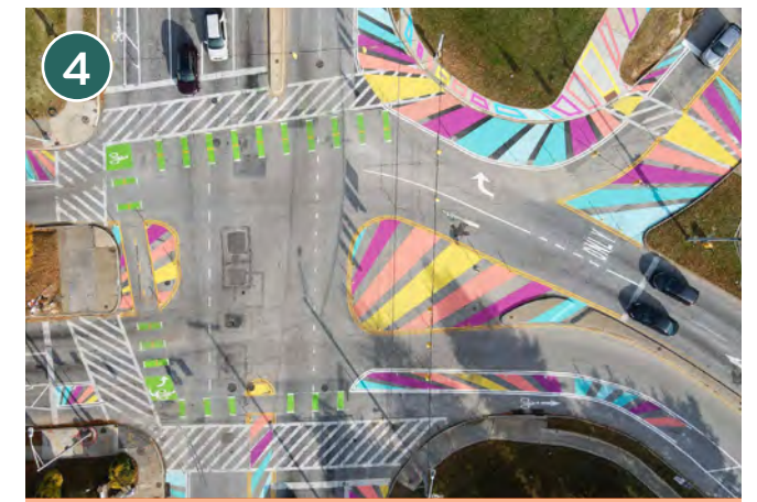
Intersection improvements near Lake Montebello
